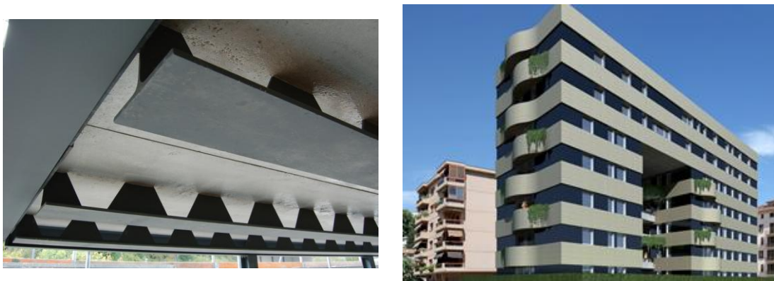
Figure 11 – Slab elements used for the enlargement of a store in Kanton Aargau (Switzerland) (left) and CAD-modell of a residential building under construction in Lugano (Switzerland) with 7 floors using the novel type of composite slab system (right)
