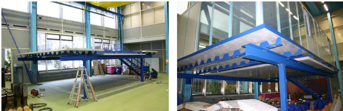
Figure 11 – New platform built using the novel type of composite slab system for a work space located in the ETH testing laboratory
